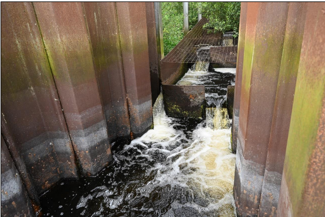
Plate 2 Non-functional fish pass at Termonbarry Weir.
