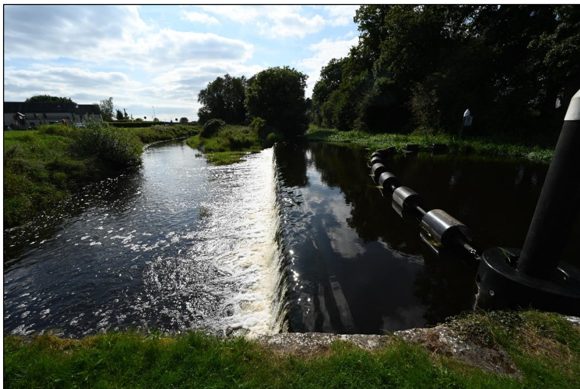
Plate 3 Navigational Weir on the River Camlin at Cloondara. One of the migration barriers in the catchment.
